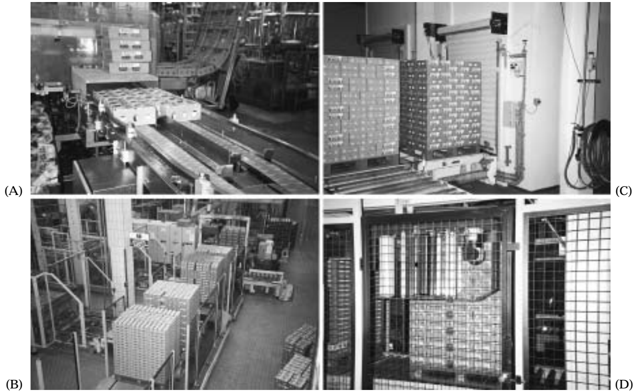
Fig. 3.66 On-site automated handling of packaged yoghurt at the Müller factory in the U.K. A, Nesting yoghurt cups in cardboard boxes; B, palletising the cardboard boxes; C, quick chill cooling in a tunnel; D, plastic overwrap of pallet.
